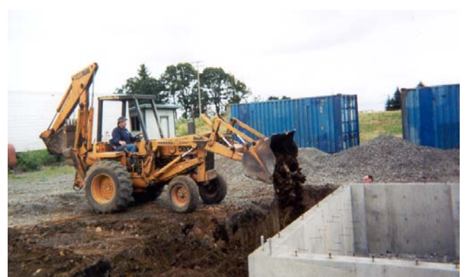
Backfilling around foundation
