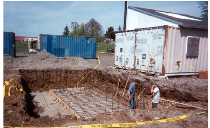
Tower foundation goes in
